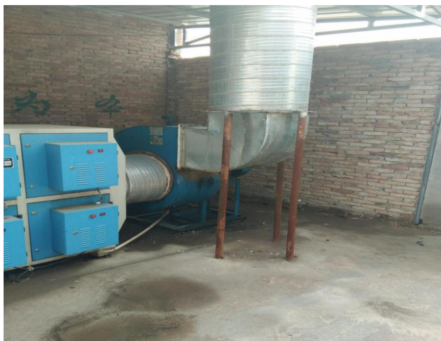
风机加设减震垫、软性接头、隔声罩
